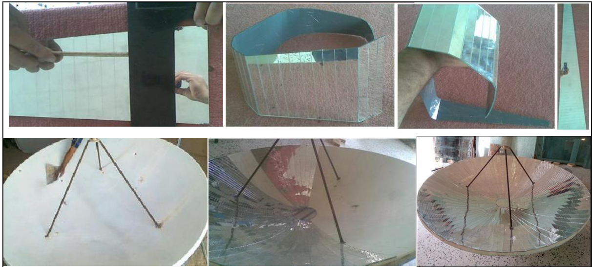
Figure 4. Fabrication process of the parabolic dish solar concentrator
