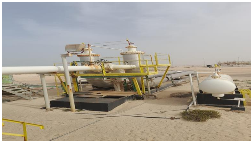
Figure 3. Bi-directional prover
