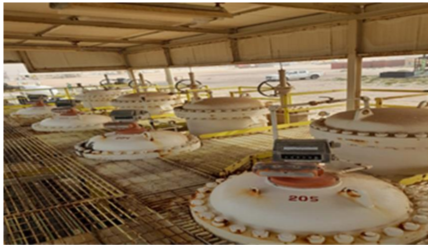
Figure2. Positive Displacement flow meter
