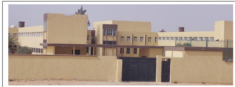
Figure 2, Two Floor Building of Jaref Elementary School
